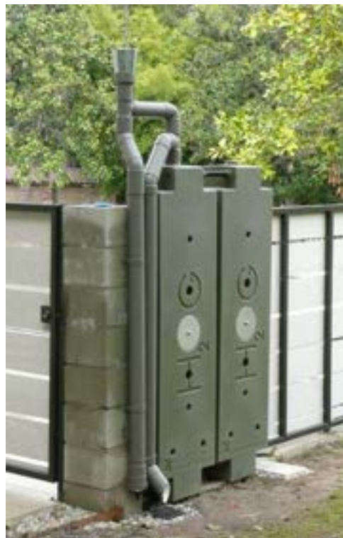
Hog System Cisterns
